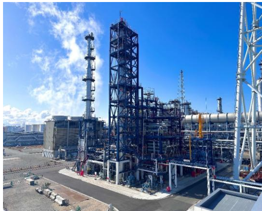
The completed SAF production line (on the premises of Cosmo Oil's Sakai Refinery)
