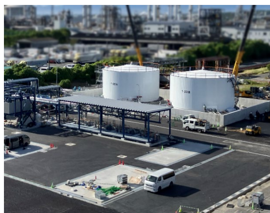
Facility for receiving used cooking oil as feedstock for SAF (on the premises of Cosmo Oil's Sakai Refinery)
