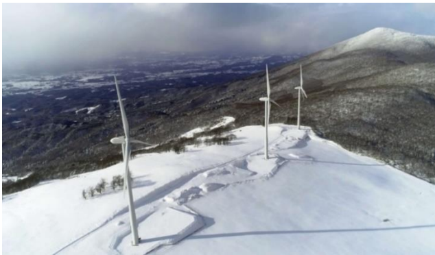
Himekami Wind Park
