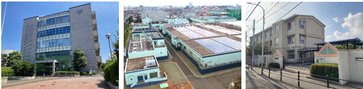
Facilities to which Cosmo Oil Marketing will newly supply renewable energy-derived electricity (From left: Sakai City Waterworks and Sewerage Bureau Headquarters Main Building, Sambo Water Recycle Center, municipal elementary school)
